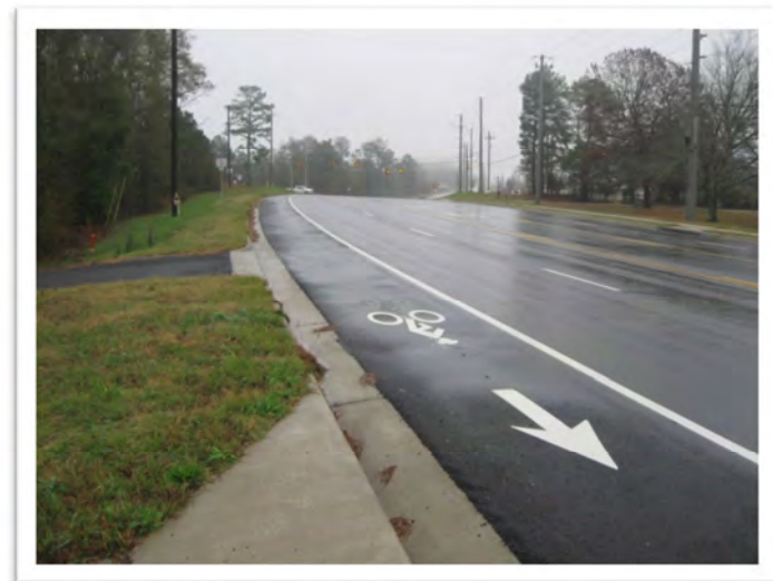
Bike Lane located on Frederick Road, Opelika, Alabama
