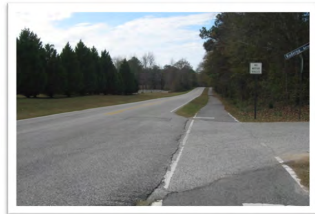
Sidepath Parallel to Wire Road, Auburn, Alabama
